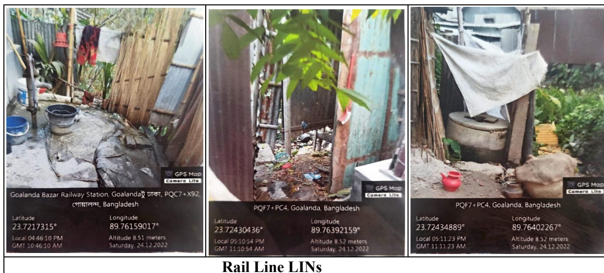
Figure IV.3: Existing Situation at Rail Line LIN
